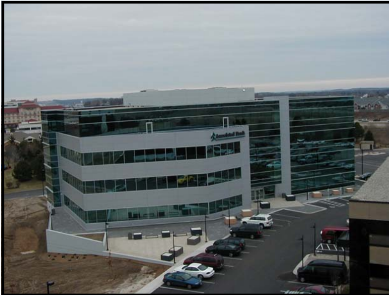
8040 Excelsior Drive exterior is completed. All that is waiting is some warm weather to finish the landscaping.
