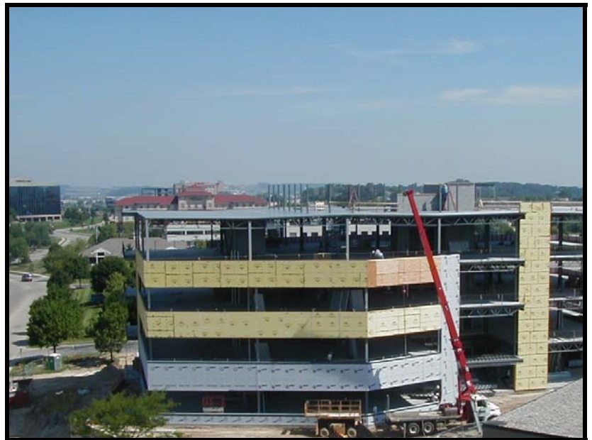
8040 Excelsior Drive will have the aluminum panels and glass installed soon.
